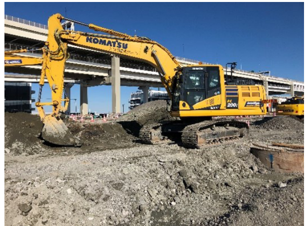
写真-8 ICT 建機施工状況
